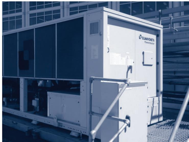
Local systems are generally used to serve a single zone or small proportion of a building, usually cooling the immediate space where they are located; they are not linked to a centralised air handling system. Local systems are often used to provide comfort cooling and are employed for cooling spaces which have a different cooling schedule from the rest of the building i.e. server rooms.
